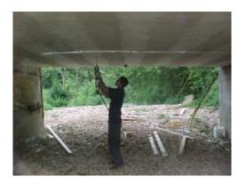
a) Crack Sealed Previous to Injection
