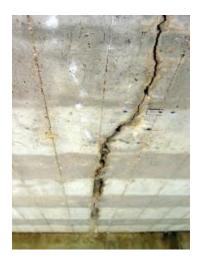
Figure 1-3 - Soffit Slab Longitudinal Crack
